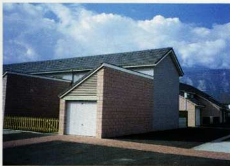
Lisse 19 - HLM Villard Bonnot 38 - Cabinet Eole
