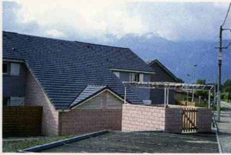
Lisse 19 - HLM Villard Bonnot 38 - Cabinet Eole
