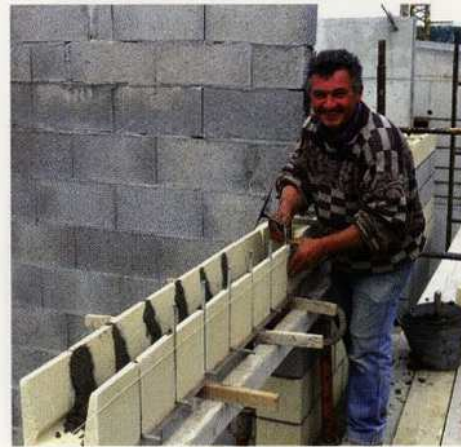
Lisse 19 - Montage Linteaux Ecole Chavanoz- 38 - Cabinet Azur
