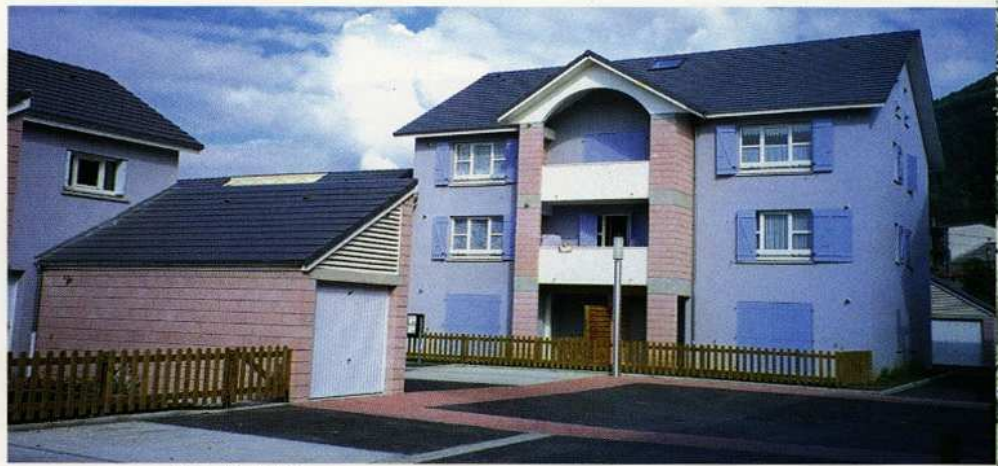
Lisse 19 - HLM Villard Bonnot 38 - Cabinet Eole
