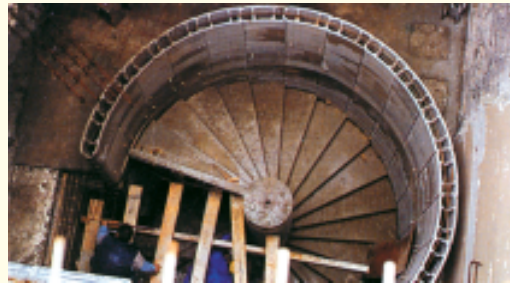
Réhabilitation - Paris - Lancuit
